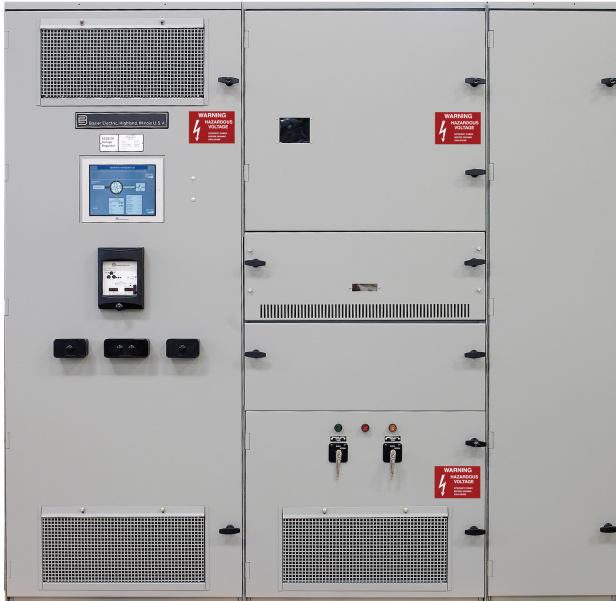
Figure 3: DECS-2100 Digital Excitation Control System
