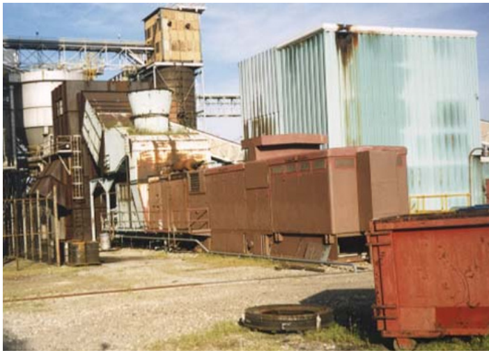
Figure 1: Combustion Turbine Generator
